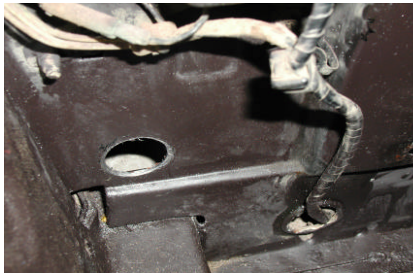
Fig. 33 Hole drilled in lower radiator support
